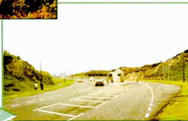
View of the toll collection point, located on the approach roads to the bridge on the mainland.
