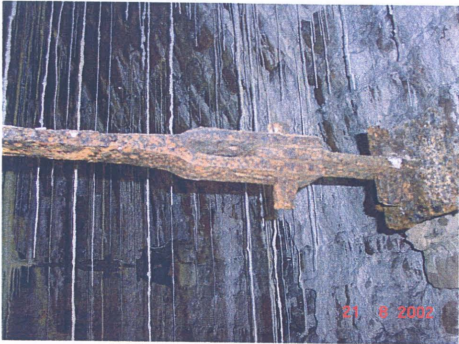
Examples of the internal ironwork.
