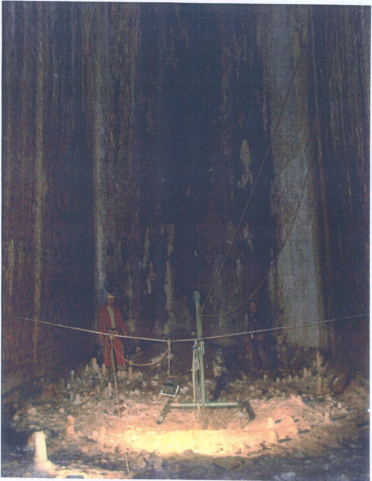
Inside one of the chambers on the Leigh Woods side.
