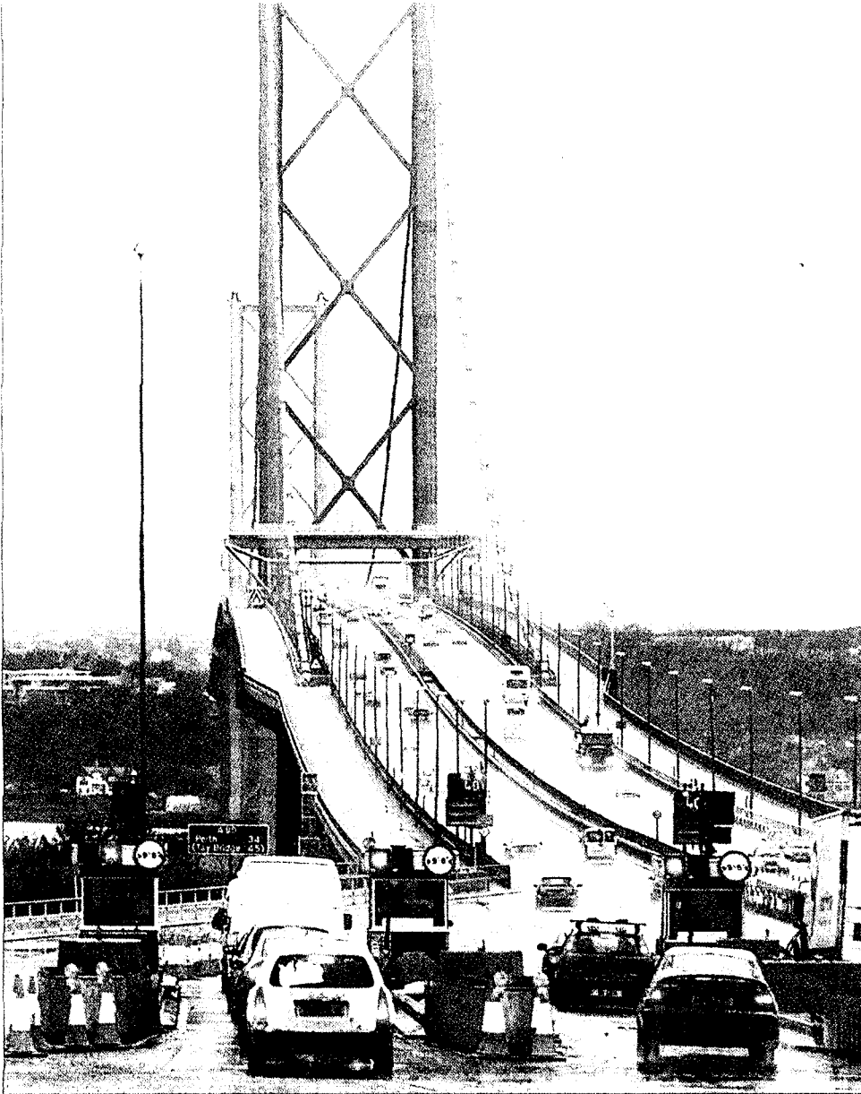
Cones channel traffic during alterations to the Forth Bridge toll booths.
